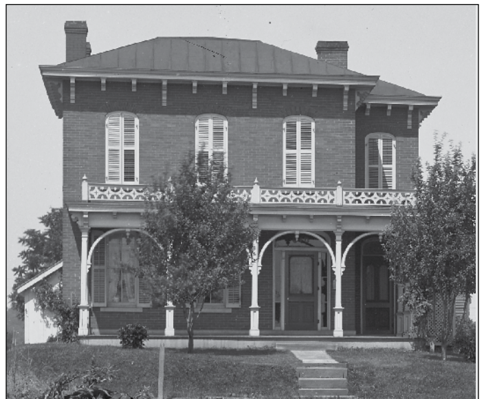
An aerial shot of progress on the replacement of the roof of the Mabel Hartzell Historical Home of the Alliance Historical Society. Right: The Mabel Hartzell House c.1890, with a standing-seem metal roof. This photograph was evidence to the History Fund's grant review committee that the Society had "done its homework" and chose a standing-seem roof in efforts to show the house when its namesake lived there. Images courtesy the Alliance Historical Society.
