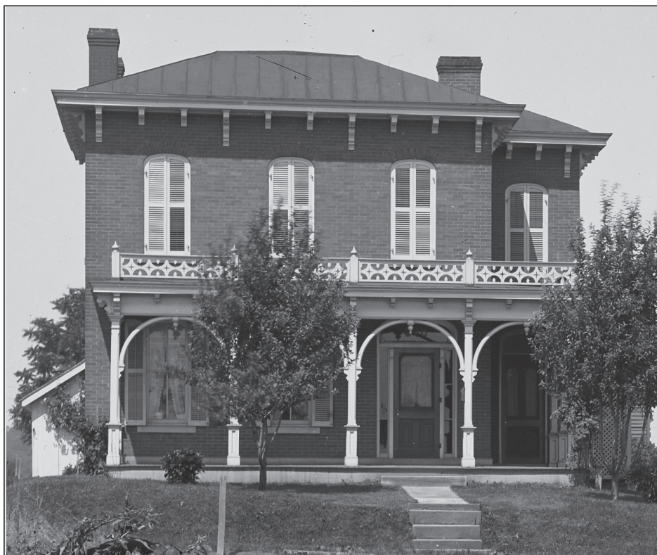
The house at 840 N. Park Ave., Alliance that would become the Mabel Hartzell Historical Home. This photo, c. 1900, and others proved that the house had a standing-seam metal roof during its period of significance and that the new roof is historically accurate.
