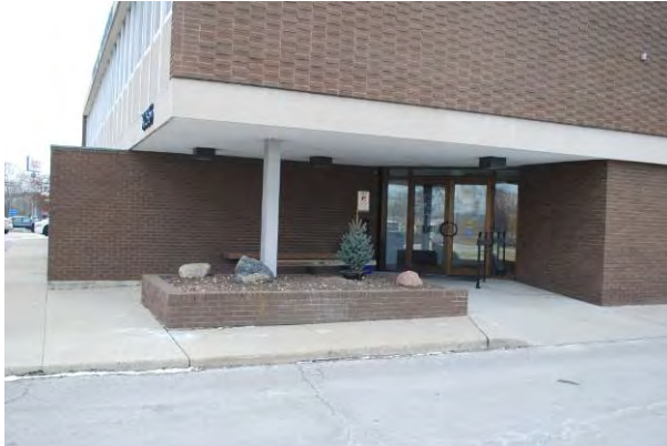
Corner recessed with planter and wing wall Trotwood Government Center (1970) 3035 Olive Rd., Trotwood MOT-05469-08
