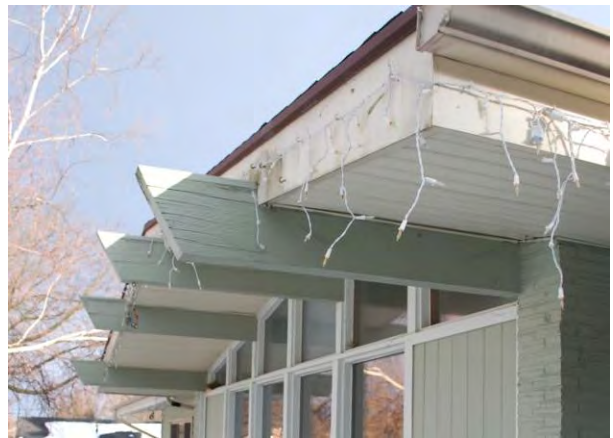
Exposed roof beams 396 Highland Terr., Kettering (1960) MOT-05545-06
