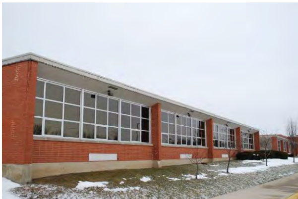
Multiple brick stacked bond Fairmont East High School (1962) 3000 Glengarry Dr., Kettering MOT-05491-06
