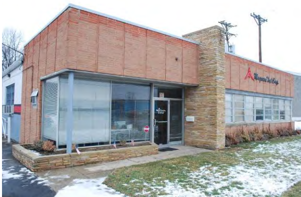
Vertical pier at entrance General Diaper Service (1955) 1407 Stanley Ave., Dayton MOT-05506-48
