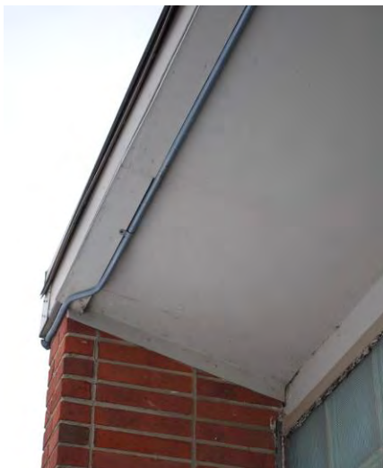
Continuous projecting - thin Rolling Fields Intermediate School (1955) 2900 Acosta St., Kettering MOT-05490-06
