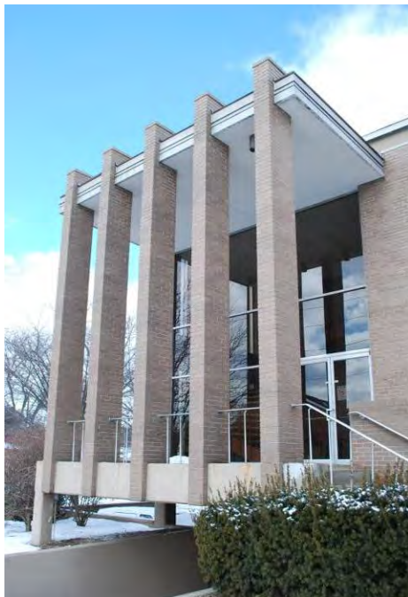
Multi-story entrance with projecting canopy 135 W. Dorothy Ln., Kettering (1963) MOT-05499-06
