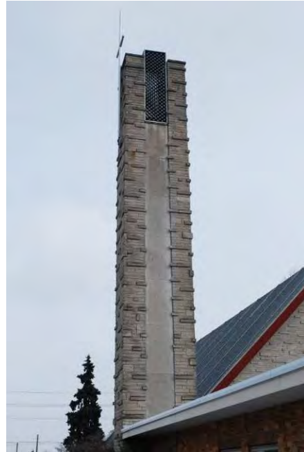
Tower with projecting elongated units Central Christian Church (1957, 1962) 1200 Forrer Blvd., Kettering MOT-05504-06
