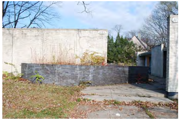
Planter wall at entrance Rothenburg Medical Building (1963) 1131-33 Salem Ave., Dayton MOT-05258-42
