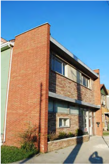
Elongated brick offset bond terminating façade 1711 E. Third St., Dayton (ca. 1960) MOT-05269-57
