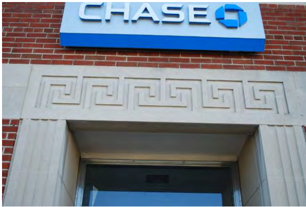
Ornamental cast stone - relief Winters National Bank & Trust (1955) 3703 N. Main St., Dayton MOT-05341-40
