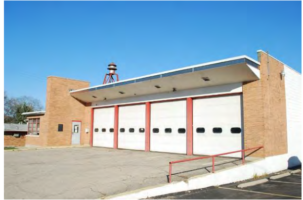
Continuous above overhead doors Harrison Twp. Fire Station #94 (1958) 5190 Markey Rd., Dayton MOT-05337-09
