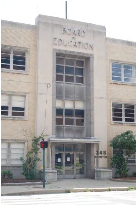
Vertical emphasis Board of Education Building (1954) 348 W. First St., Dayton MOT-05150-15
