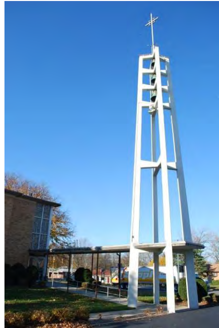
Bell tower with canopy
