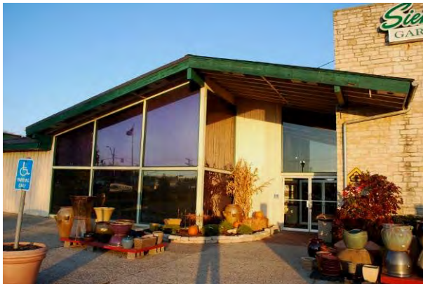
Low pitched gable with projecting eaves Siebenthaler Garden Center (1960) 6000 Far Hills Ave., Centerville MOT-05218-03
