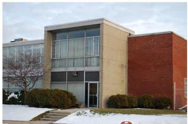
Vertical emphasis - projecting with concrete wing walls Globe Industries, Inc. (1954) 1784 Stanley Ave., Dayton MOT-05509-48
