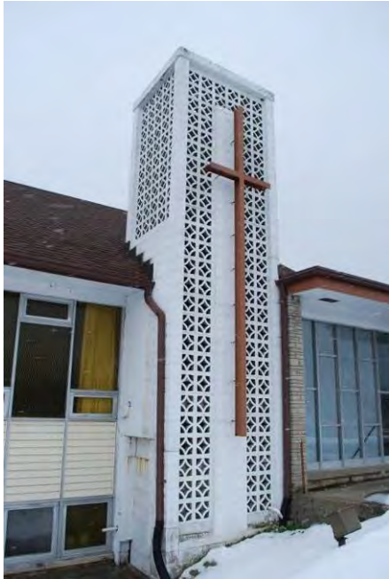
Tower with ornamental block Calvary Brethren Church (1962) 2850 E. Dorothy Ln., Kettering MOT-05489-06
