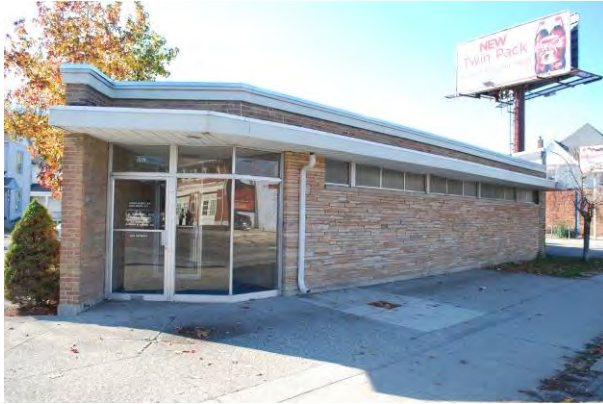
Continuous above entrance and windows with return 1501 N. Main St., Dayton (1957) MOT-05343-42
