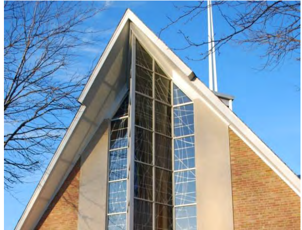
Prow - stepped Trinity Evangelical Lutheran Church (1963) 6540 N. Main St., Dayton MOT-05331-09
