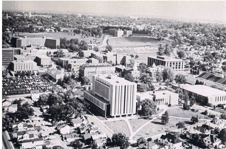
1975 Aerial view showing the extent of mid-20 th -century buildings added to the campus. Roesch Library is in the center. (Historic Image 7)
