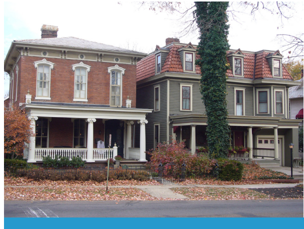
Porches along Wheeling Street, Lancaster
