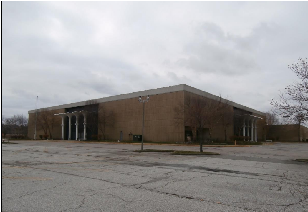
Plate 3. Euclid Square Mall (CUY 1104522), constructed in 1976, Euclid. Currently mostly vacant with no remaining retail stores; however, this former anchor store end retains its original entry columns.
