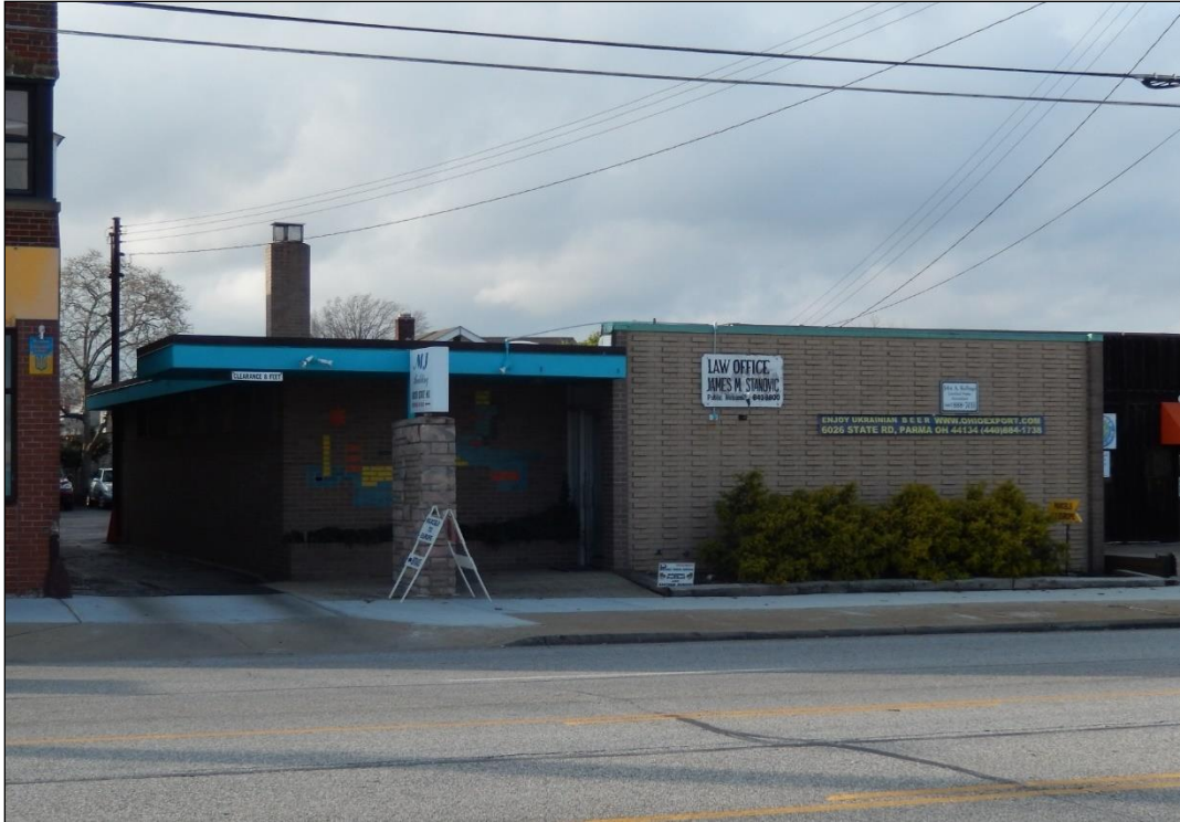
Plate 7. MJ Building (CUY 1145417), constructed in 1956, 6020 State Rd., Parma. The building was advertised as ideal for small medical offices, and currently houses law and accountant offices.
