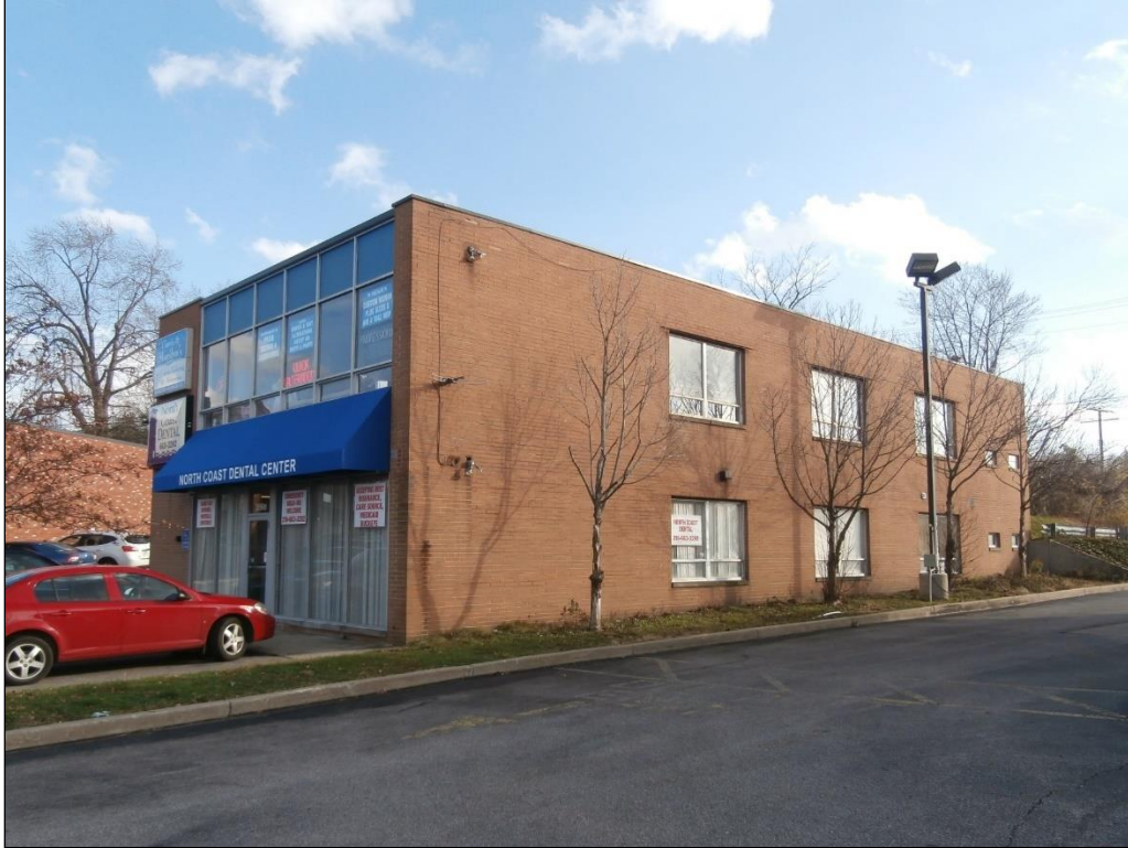
Plate 5. Small retail store (CUY 1134624), constructed in 1964, 20508 Southgate Park Blvd., Maple Heights. The building retains most original materials.
